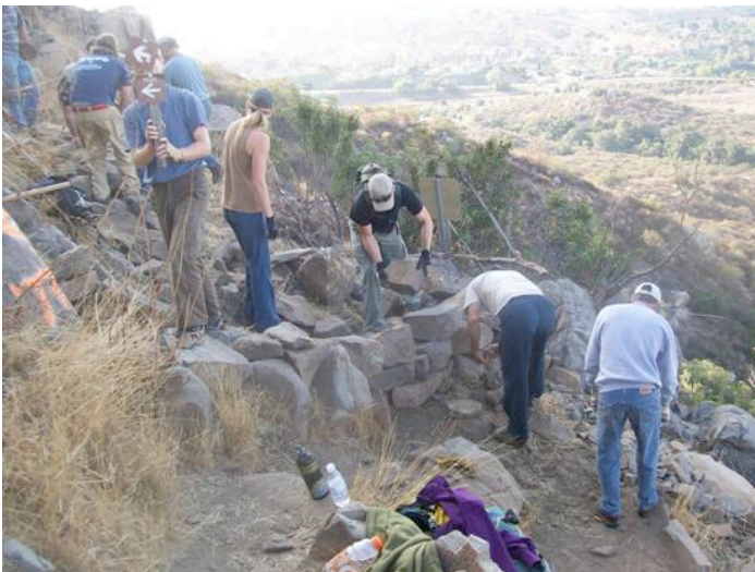
Members of Allied Climbers erecting a dry-stack wall
